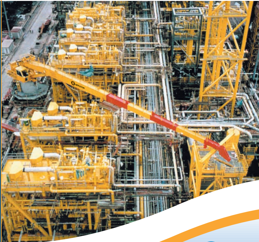
Floating Production Storage Offloading (FPSO) Maintenance Crane
